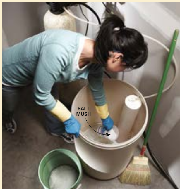
Scoop out the mush at the bottom of the tank, then pour in hot water to dissolve the rest before regenerating the system.
