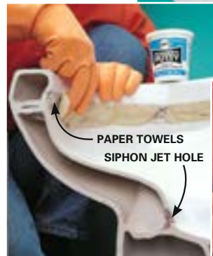
B SEAL the rinse holes
