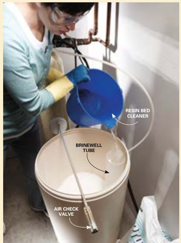
Pour diluted resin cleaner into the brinewell tube. Lift out the air check valve (or brine valve assembly) and clean it in warm water.
